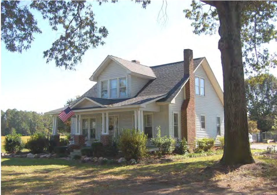
Plate 178. Percy and Mynette Strother House, House and Setting, Looking Southeast.
