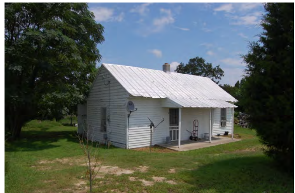
No. 48 House (PIN 16082881112), 5205 Holland Church Road, Garner Vicinity, Wake County
