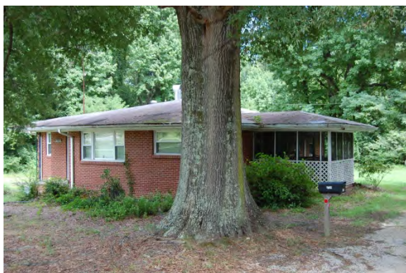
No. 25 House (PIN 0689441793), 8729 Lake Wheeler Road, McCullers Crossroads Vicinity, Wake County
