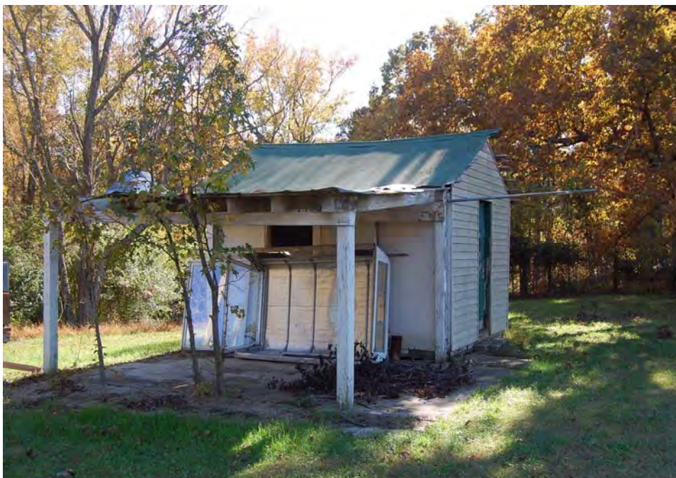
Plate 84. G. L. Pierce House, Storage Shed West of House, Looking South.
