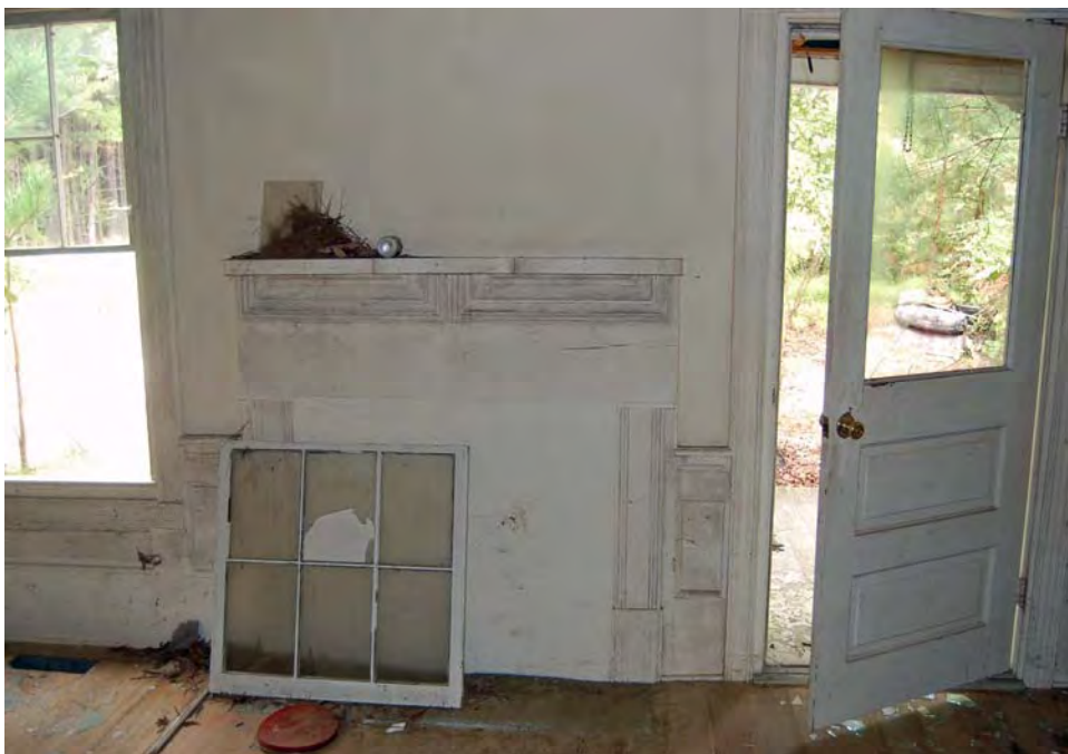
Plate 65. Penny House, Interior, North Room, Mantel and Door to Porch.
