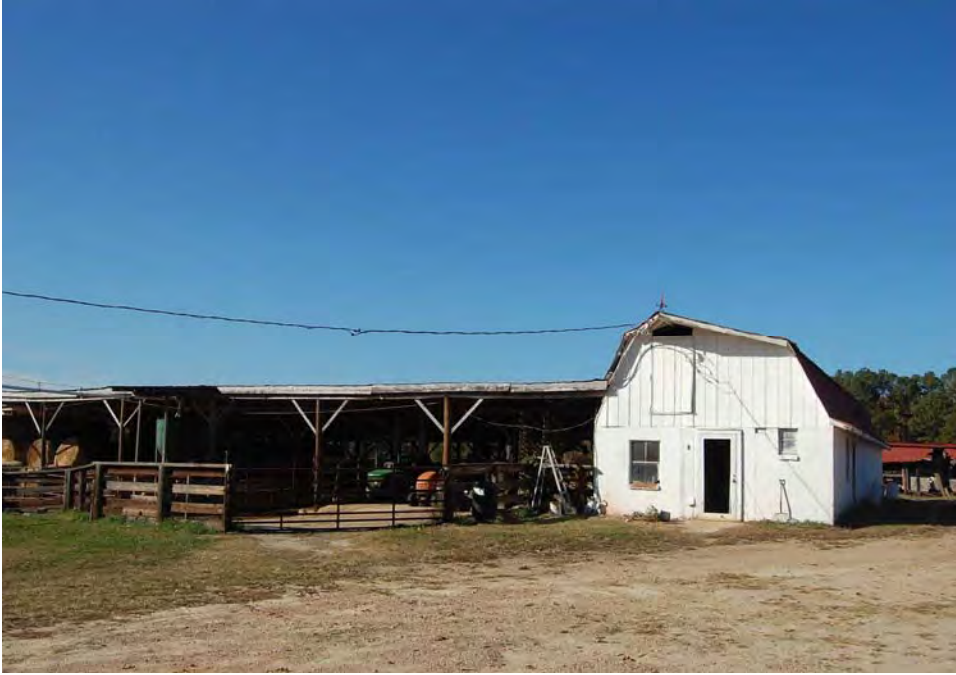
Plate 106. Pierce Farm, Dairy Barn, Looking North.
