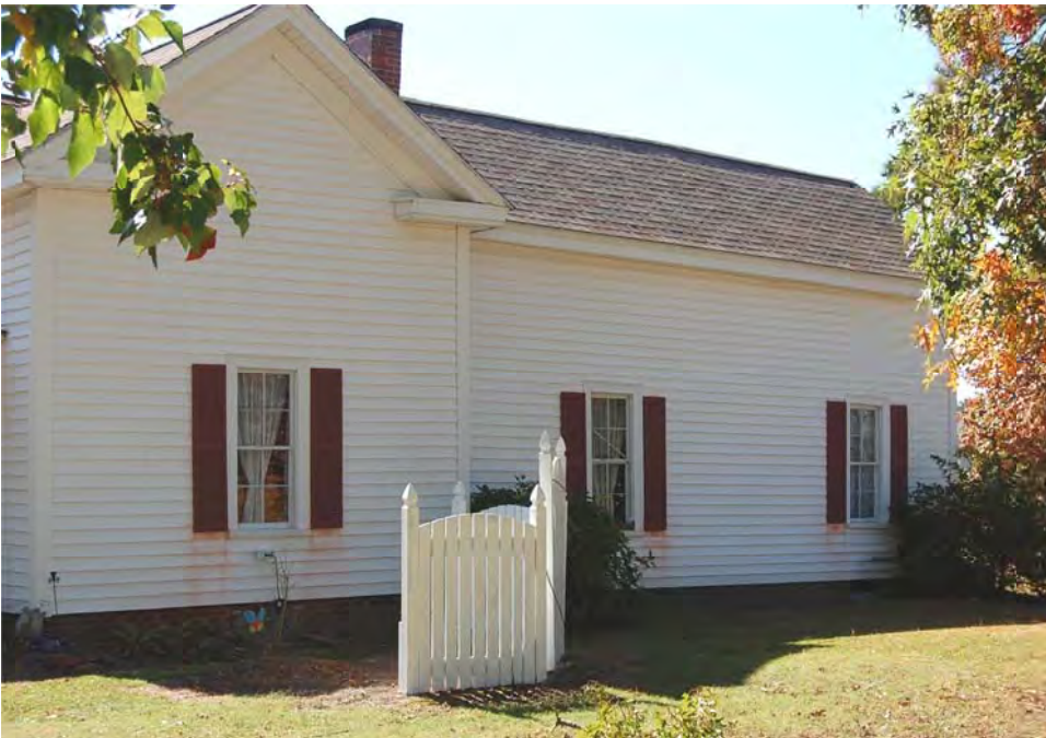
Plate 247. Juniper Level, House, 9114 Sauls Road (WA5733), Side (North) Elevation, Looking Southwest.
