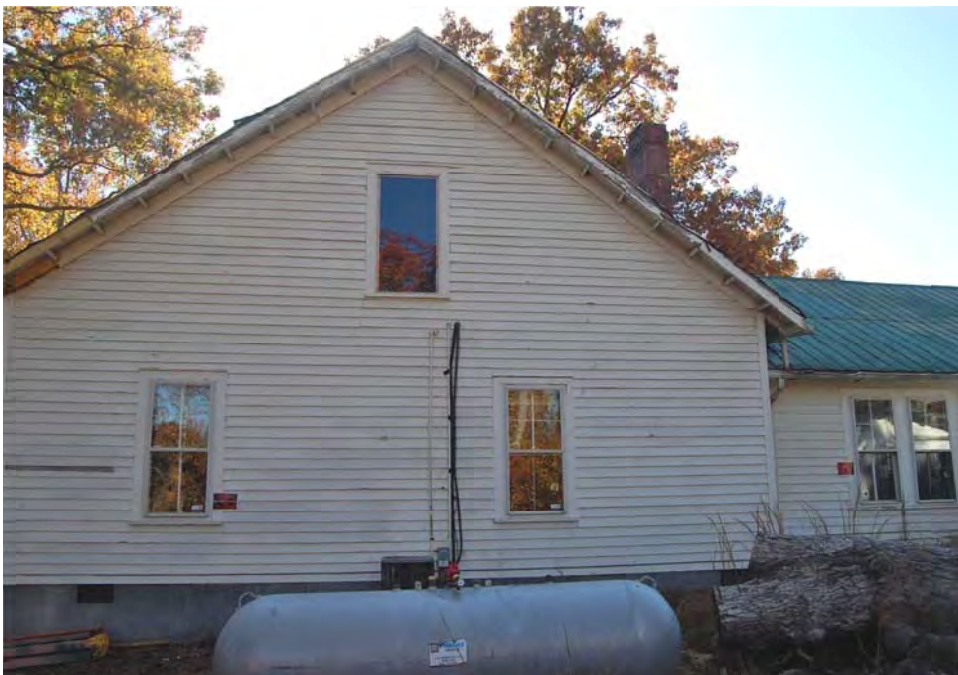
Plate 81. G. L. Pierce House, Side (North) Elevation, Looking South.
