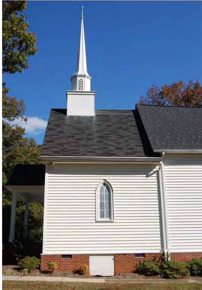
Plate 169. Wentworth Christian Church, Modern Front Addition, West Elevation, Looking East.
