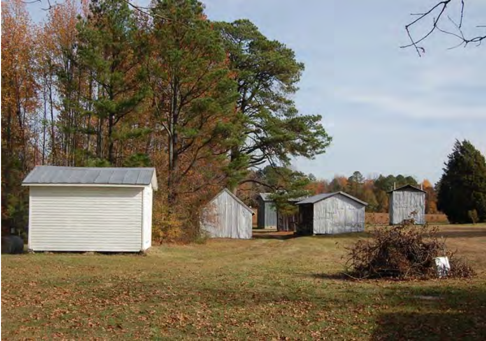
Plate 222. George Williams Farm, Storage Shed, Packhouses, Tobacco Barns, Looking East.
