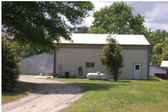
No. 177 Pope Farm (WA1968) (PIN 1743945183), 1004 Bethlehem Road Garner Vicinity, Wake County
