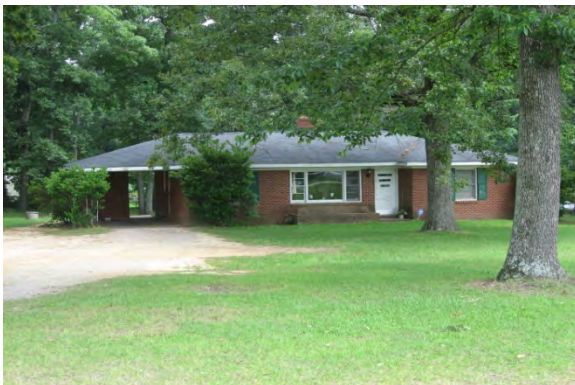
No. 185 House (PIN 0689853678), 8309 Fayetteville Road, Garner Vicinity, Wake County
