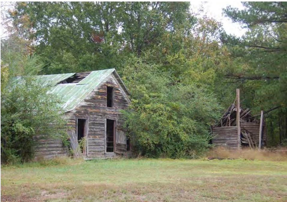
Plate 77. Baucom-Stallings House, Ruinous Barns East of House, Looking East.
