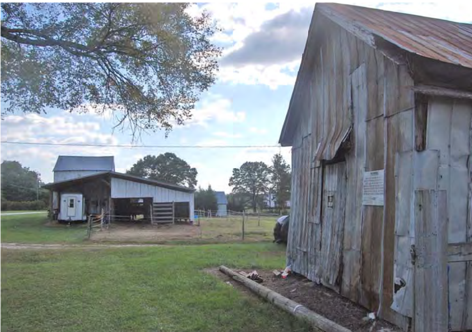
Plate 277. Jones Family Farm, Shed and Tobacco Barn, Looking South.
