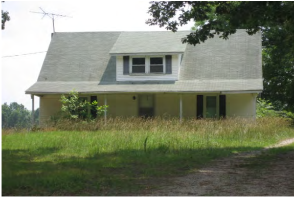
No. 182 House (PIN 0689953648), 8216 Ten Ten Road, Garner Vicinity, Wake County
