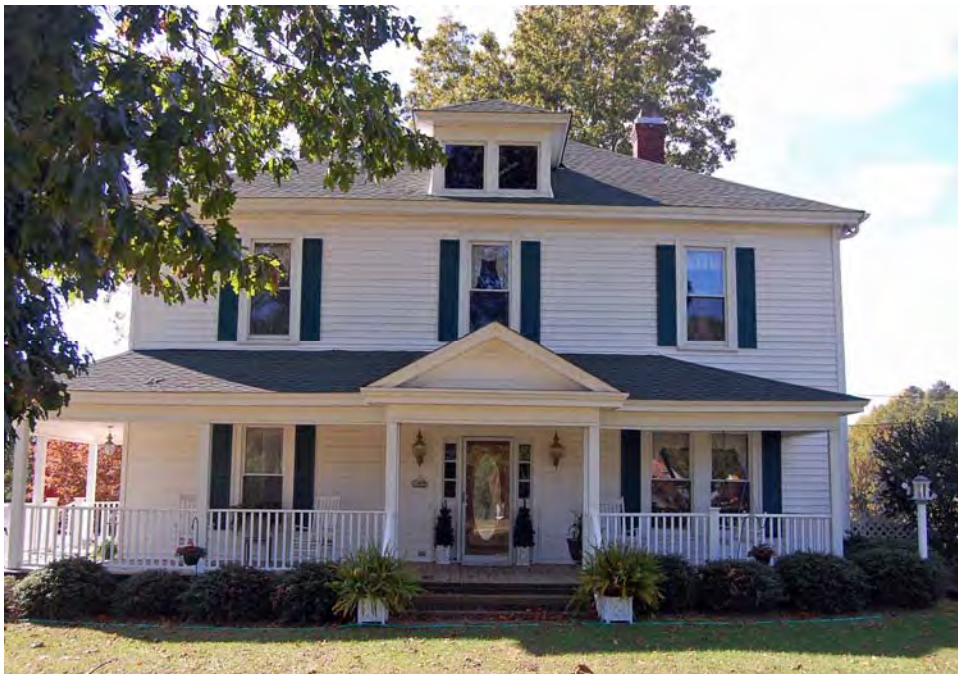
Plate 232. Samuel Jefferson Rhodes House, Façade, Looking West.
