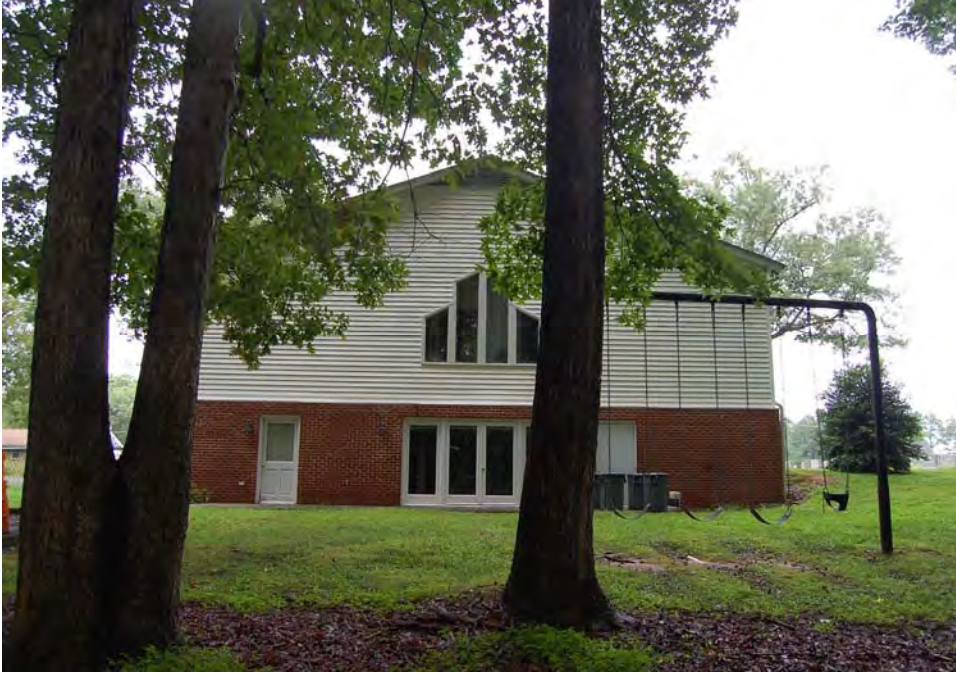
Plate 168. Wentworth Christian Church, Rear Elevation Addition, Looking North.
