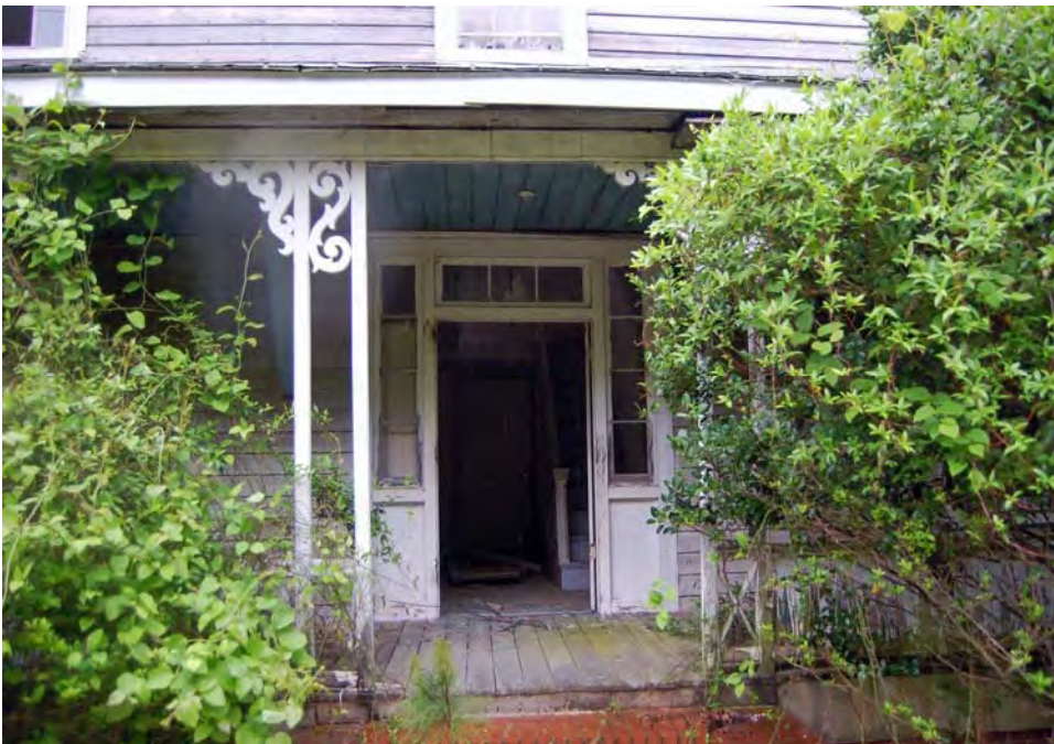
Plate 57. Penny House, Entrance and Porch Details, Looking East.
