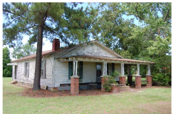
No. 19 House (PIN 0689189792, 3812 Johnson Pond Road, Apex Vicinity, Wake County
