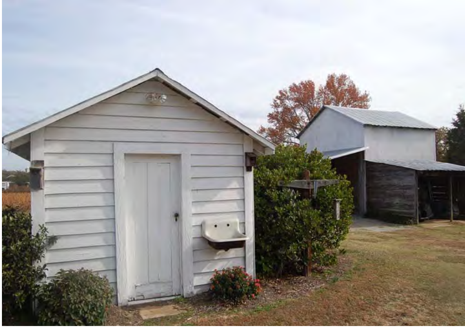
Plate 142. Bell-Pierce Farm, Eastern Tract (WA1252), Smokehouse and Packhouse, Looking Southeast.
