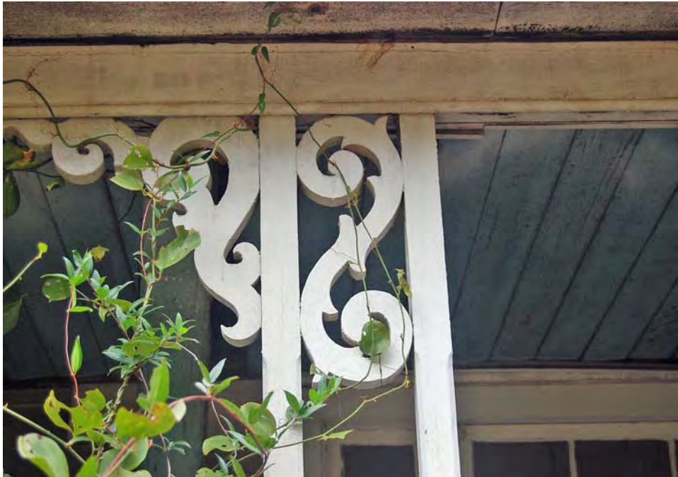
Plate 58. Penny House, Porch Detail, Looking East.
