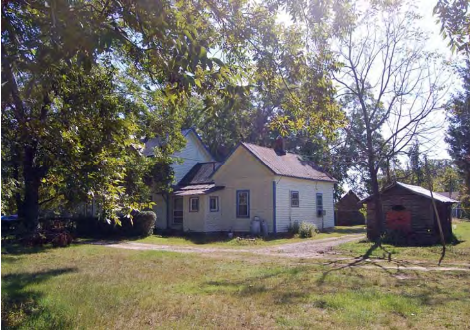
Plate 28. W. A. Gowers Farm, House, Rear Kitchen Wing and Washhouse, Looking South.
