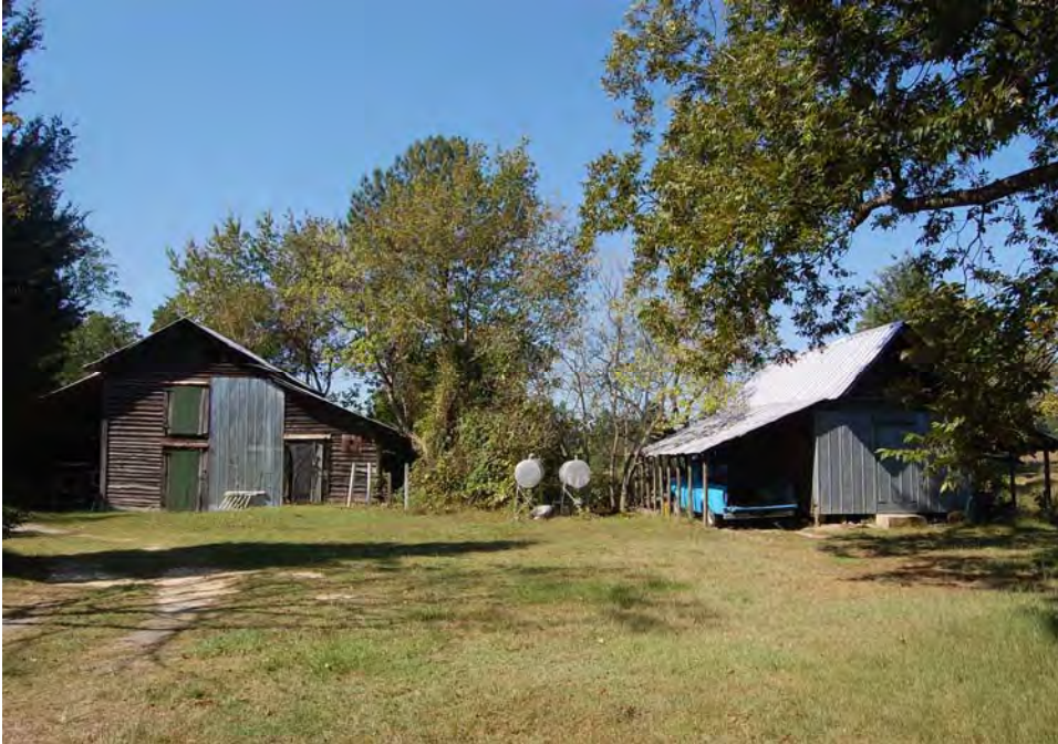
Plate 26. W. A. Gowers Farm, Packhouse and Corncrib, Looking West.
