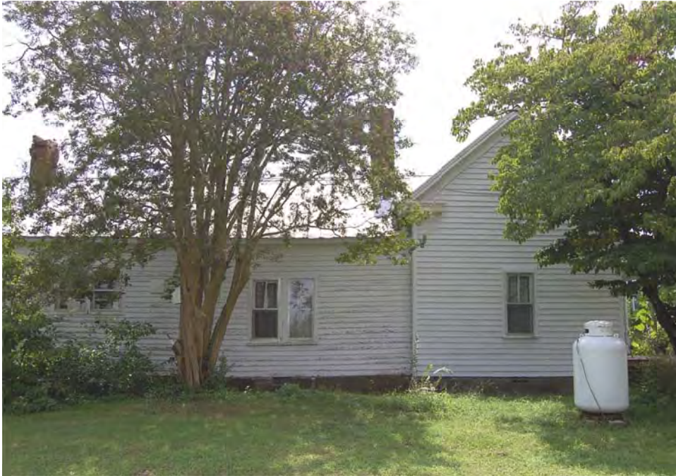
Plate 270. Jones Family Farm, House, Side (North) Elevation, Looking South.
