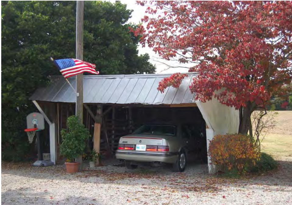
Plate 156. Bell-Pierce Farm, Western Tract, Equipment Shed/Garage, Looking West.
