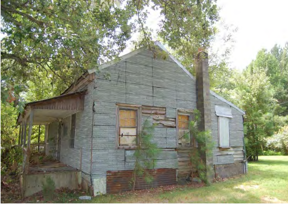
Plate 86. Wes Jones Farm, House, Side (North) Elevation, Looking South.
