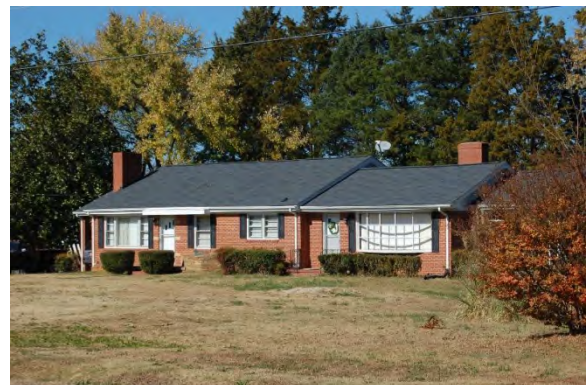
No. 195 House (PIN 1742891507), 7801 Poole Road, Garner Vicinity, Wake County
