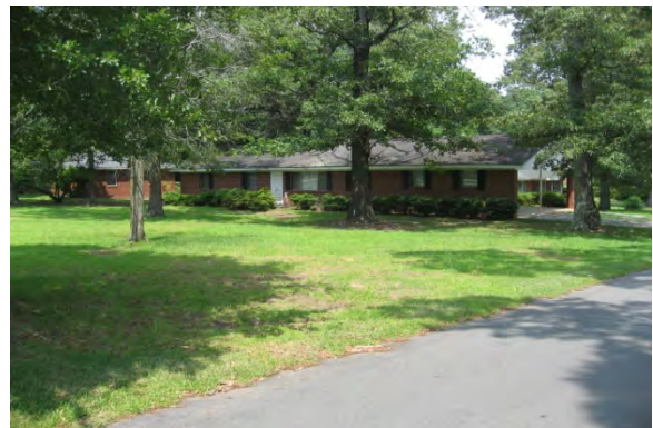
No. 186 House (PIN 0689853537), 8313 Fayetteville Road, Garner Vicinity, Wake County
