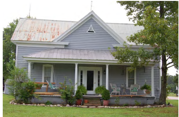
No. 31 House (WA1223) (PIN 0699422621), 9013 Fanny Brown Road, McCullers Crossroads Vicinity, Wake County
