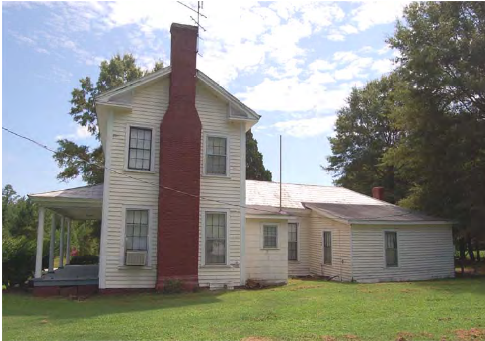
Plate 12. John B. Strain House, Side (North) Elevation, Looking South
