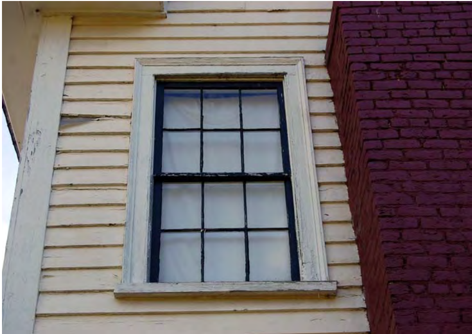
Plate 16. John B. Strain House, Window Detail, South Elevation.
