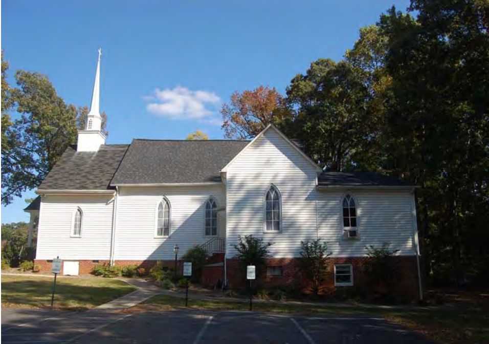
Plate 166. Wentworth Christian Church, Side (West) Elevation, Looking East.
