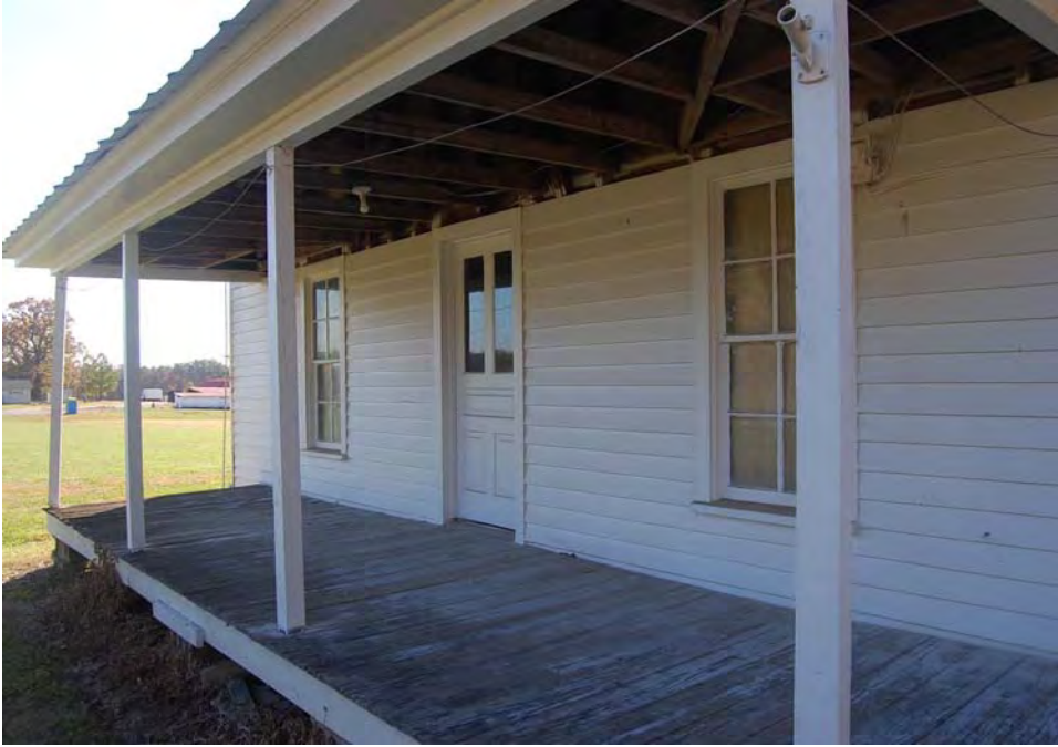
Plate 120. C. B. Sorrell House, Front Porch, Looking South.
