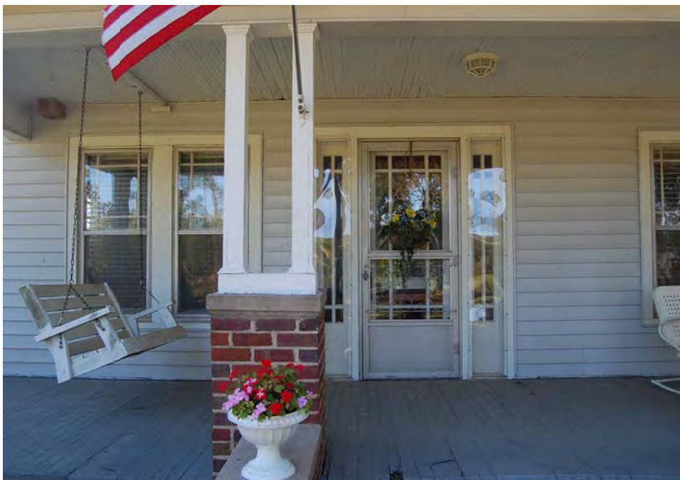
Plate 181. Percy and Mynette Strother House, Main Entrance and Porch Details.
