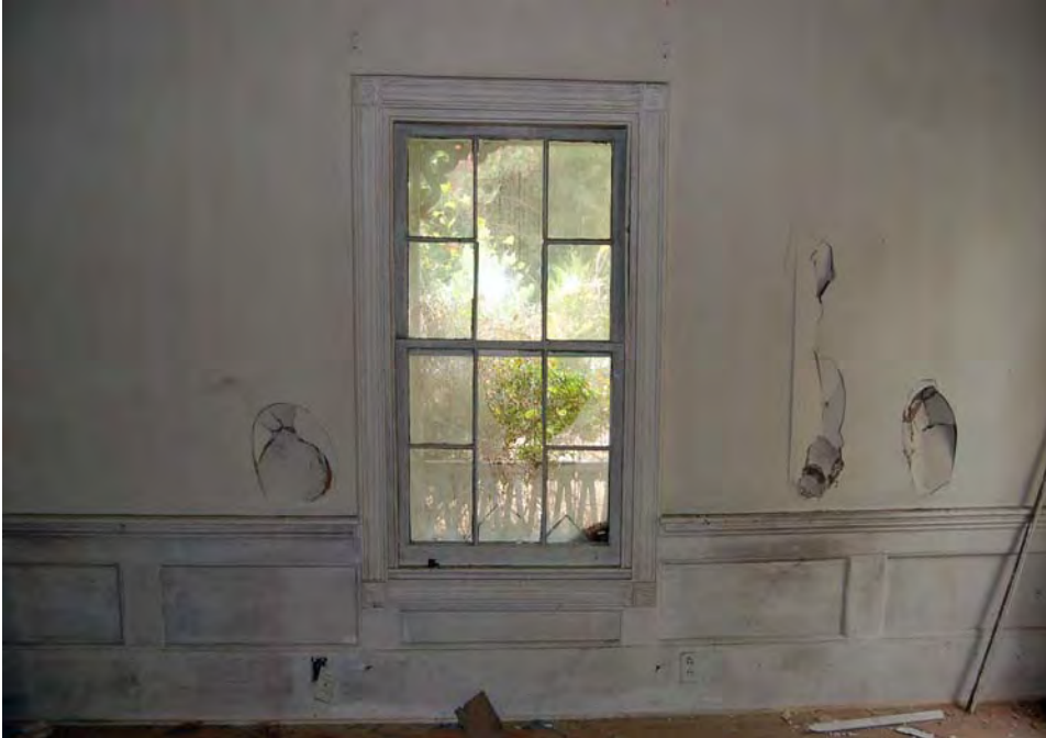
Plate 66. Penny House, North Room, Window and Wainscoting.
