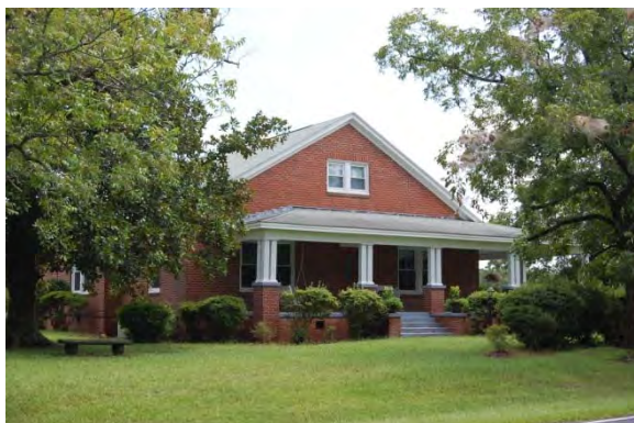
No. 52 House (PIN 1609117174), 4825 Holland Church Road, Garner Vicinity, Wake County
