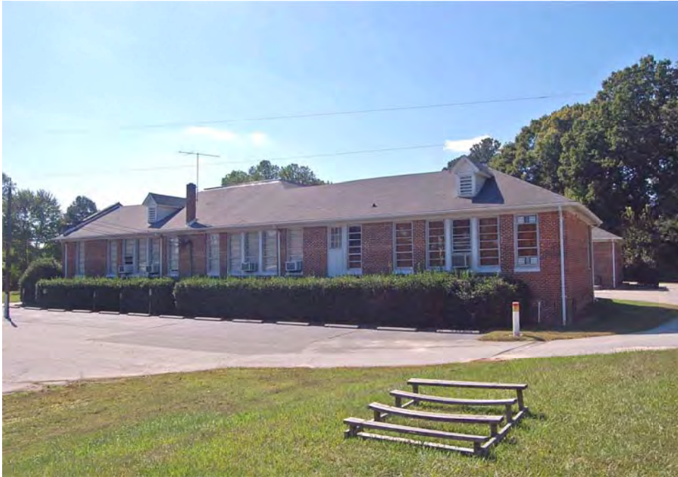
Plate 47. Mount Auburn School, East Elevation, Looking West from Gymnasium.
