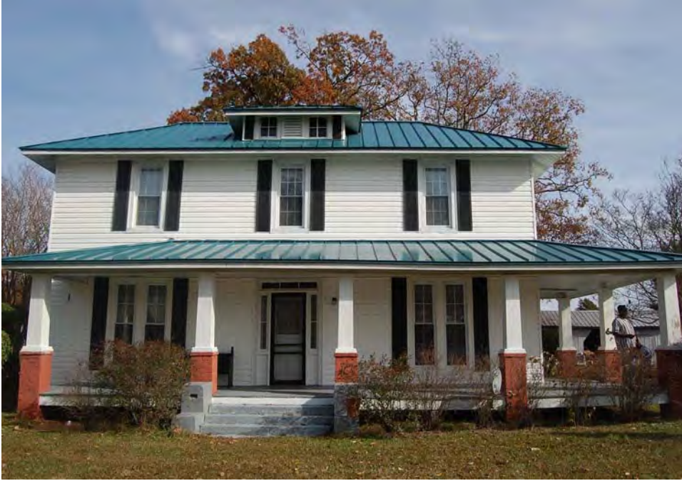
Plate 216. George Williams Farm, House Facade, Looking East.
