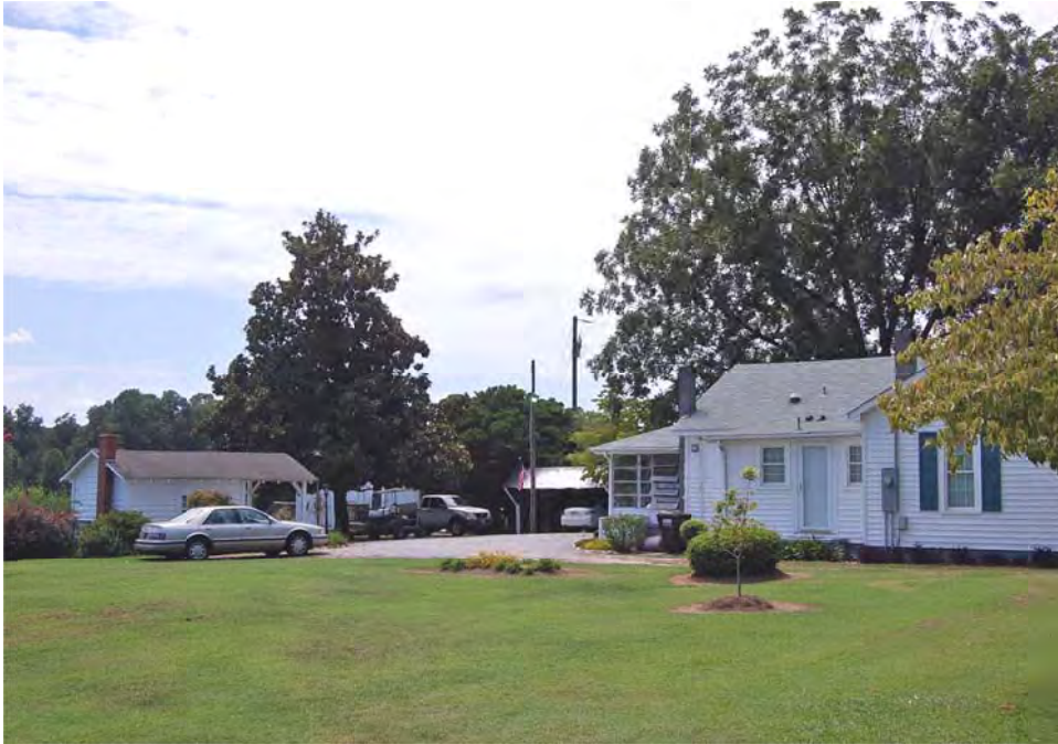
Plate 154. Bell-Pierce Farm, Western Tract, House, East Elevation, and Washhouse, Looking Southwest.
