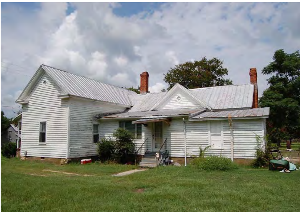
Plate 269. Jones Family Farm, House, Side (South) Elevation and Rear Ell, Looking North.
