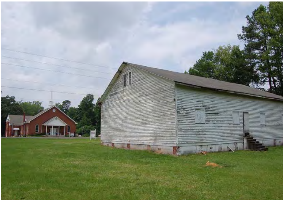
Plate 2. Panther Branch School, Looking West towards Juniper Level Baptist Church.
