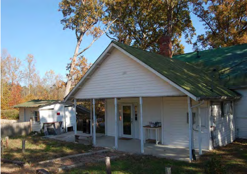
Plate 82. G. L. Pierce House, Rear (West) Elevation and Shed, Looking Northeast.
