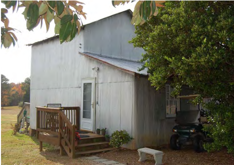
Plate 160. Bell-Pierce Farm, Western Tract, Packhouse (Now Office), Looking South.
