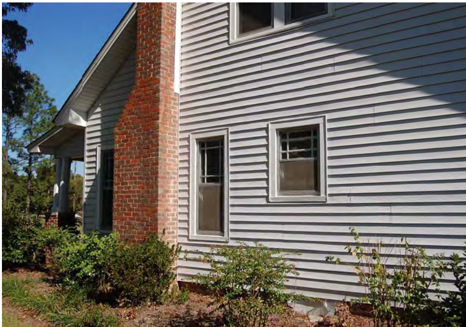
Plate 183. Percy and Mynette Strother House, Side (West) Elevation, Looking Northeast.
