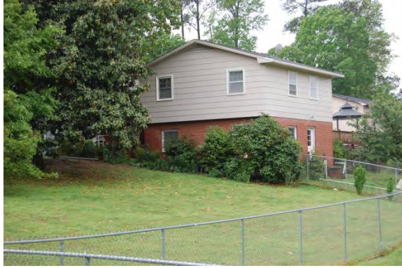
No. 139 House (PIN 1741211251) 2624 Branch Road, Garner Vicinity, Wake County
