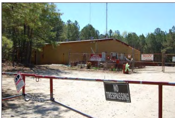
No. 84 American Metal and Parts Company Building (PIN 1730732237), 2212 US 70 Highway East, Garner Vicinity, Wake County
