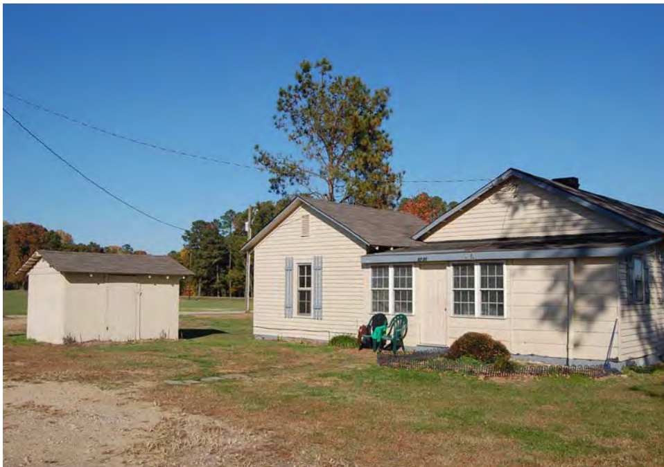
Plate 105. Pierce Farm, Pierce House (WA5695), Rear Elevation and Pump House, Looking Northeast.
