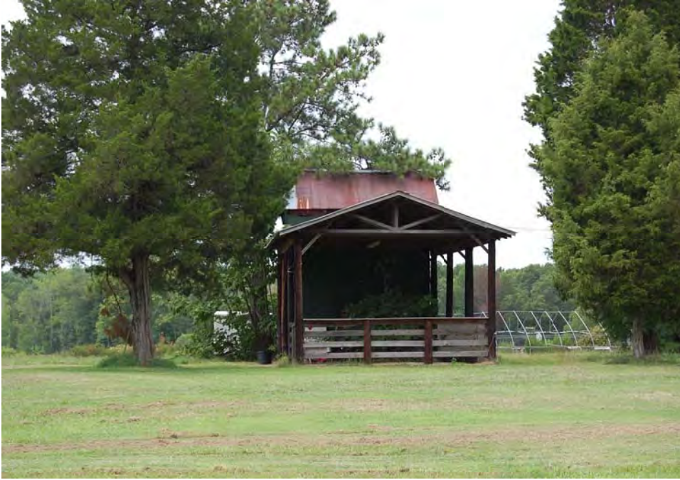
Plate 124. C. B. Sorrell House, Tobacco Barn, Looking West.
