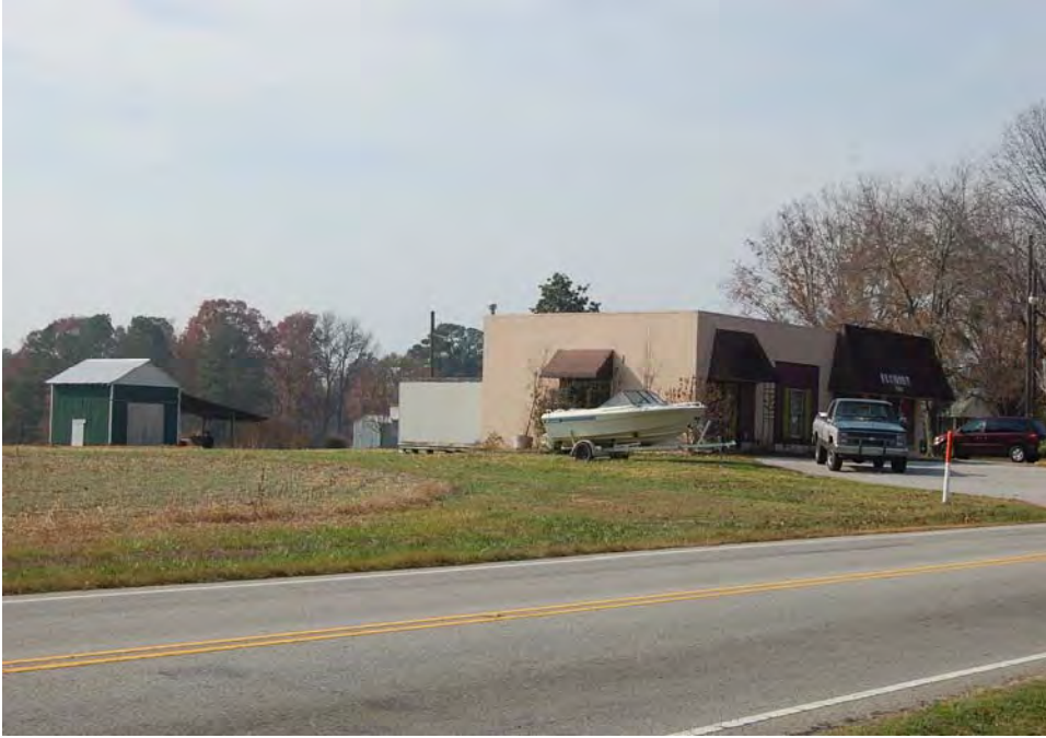
Plate 162. Bell-Pierce Farm, Western Tract, Modern Commercial Building along Ten Ten Road, Looking West.
