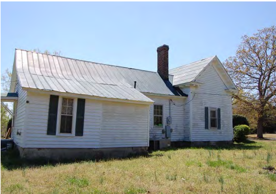
Plate 40. Gower-Johnson House, North Elevation and Rear Ell, Looking South.
