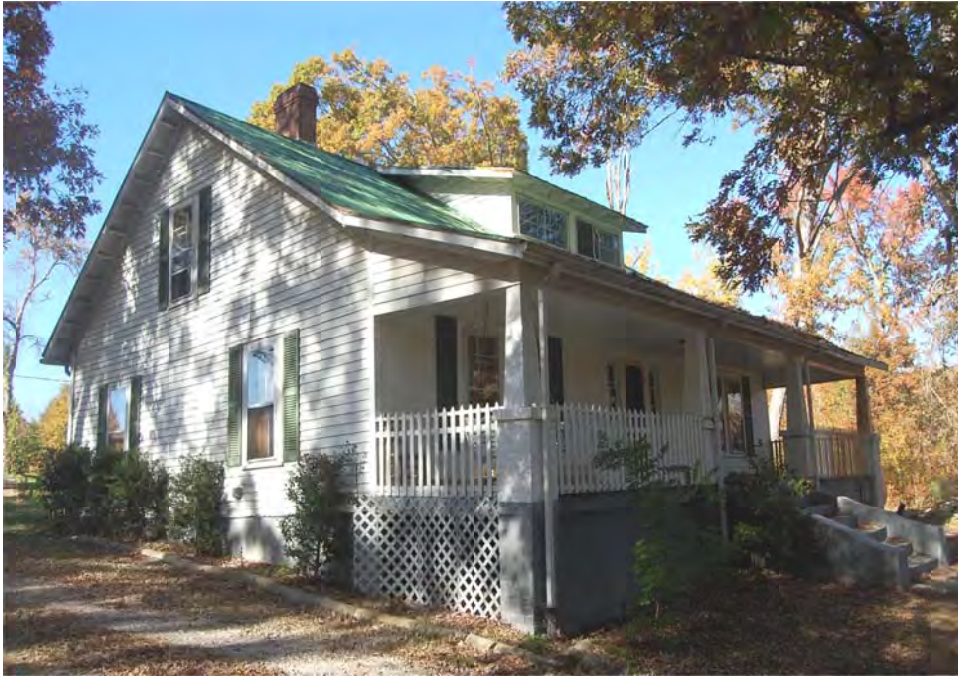
Plate 80. G. L. Pierce House, Façade (East Elevation) and Side (South) Elevation, Looking Northwest.
