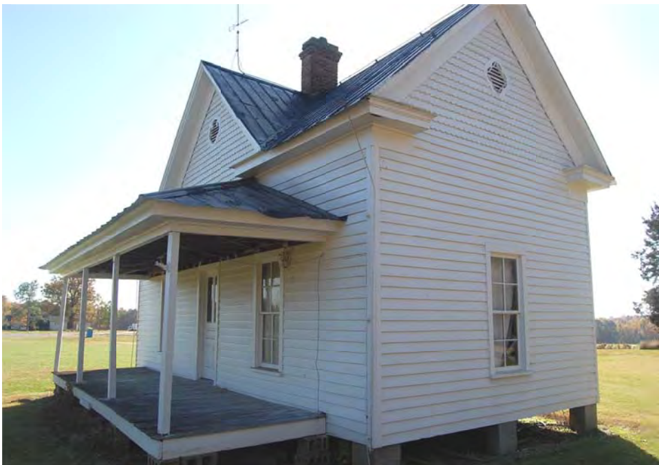
Plate 123. C. B. Sorrell House, Front (East) and Side (North) Elevations, Looking South.
