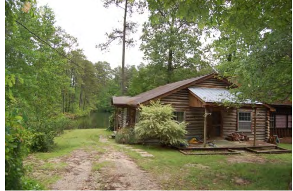
No. 158 House (PIN 1742651371) 3061 Hodge Road, Garner Vicinity, Wake County
