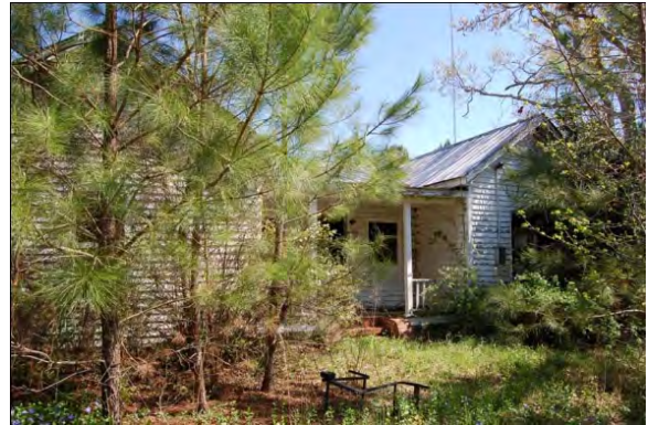
No. 116 House (PIN 1730837850), 4812 Green Garden Road, Garner Vicinity, Wake County
