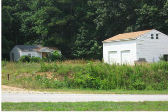
No. 187 House (PIN 0688585940), 9620 Fayetteville Road, Garner Vicinity, Wake County
