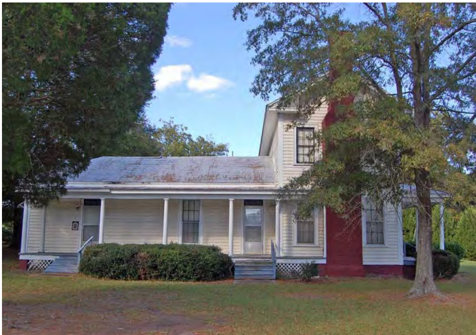
Plate 13. John B. Strain House, Side (South) Elevation, Looking North.
