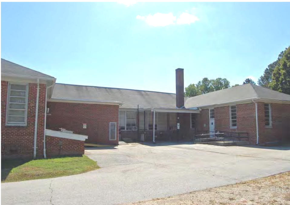
Plate 48. Mount Auburn School, Rear (North) Elevation, Looking South.
