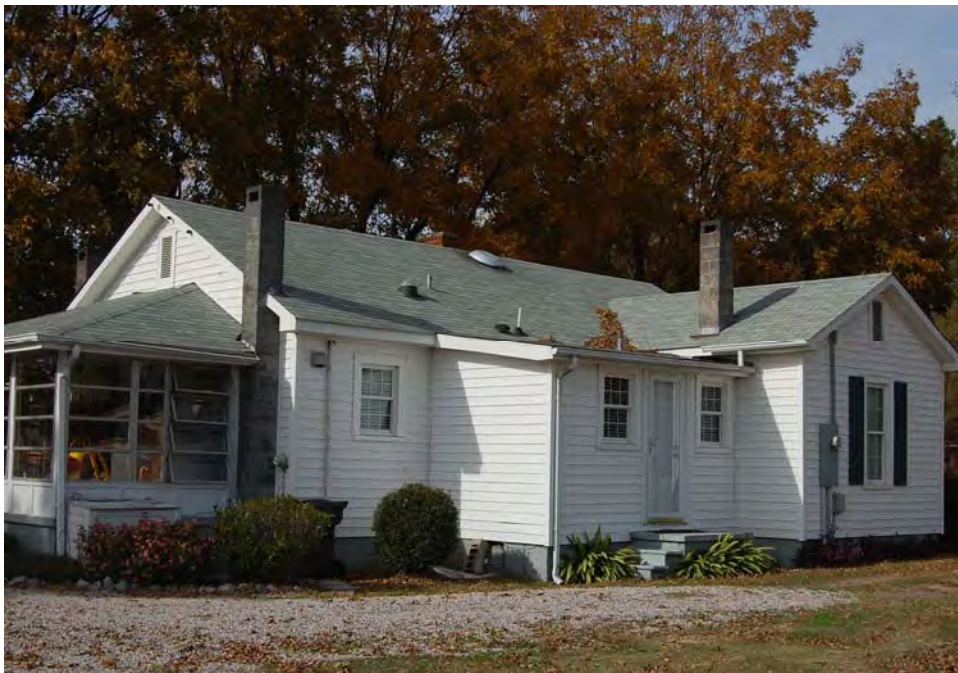
Plate 153. Bell-Pierce Farm, Western Tract, House, Side (East) and Rear (South) Elevations, Looking North.
