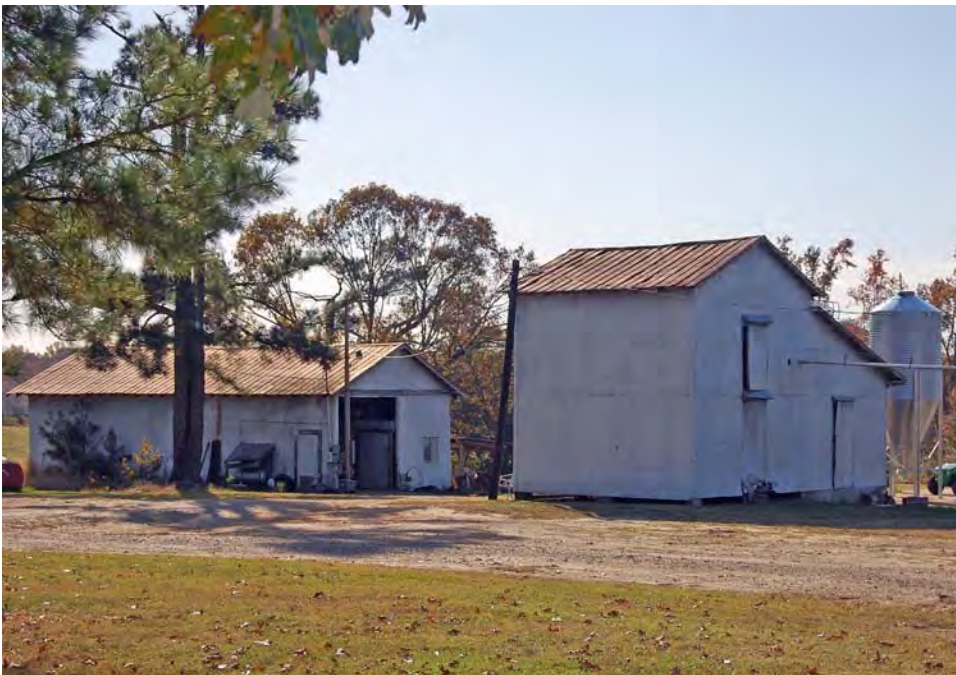
Plate 111. Pierce Farm, Packhouse and Equipment Storage Building, Looking West.
