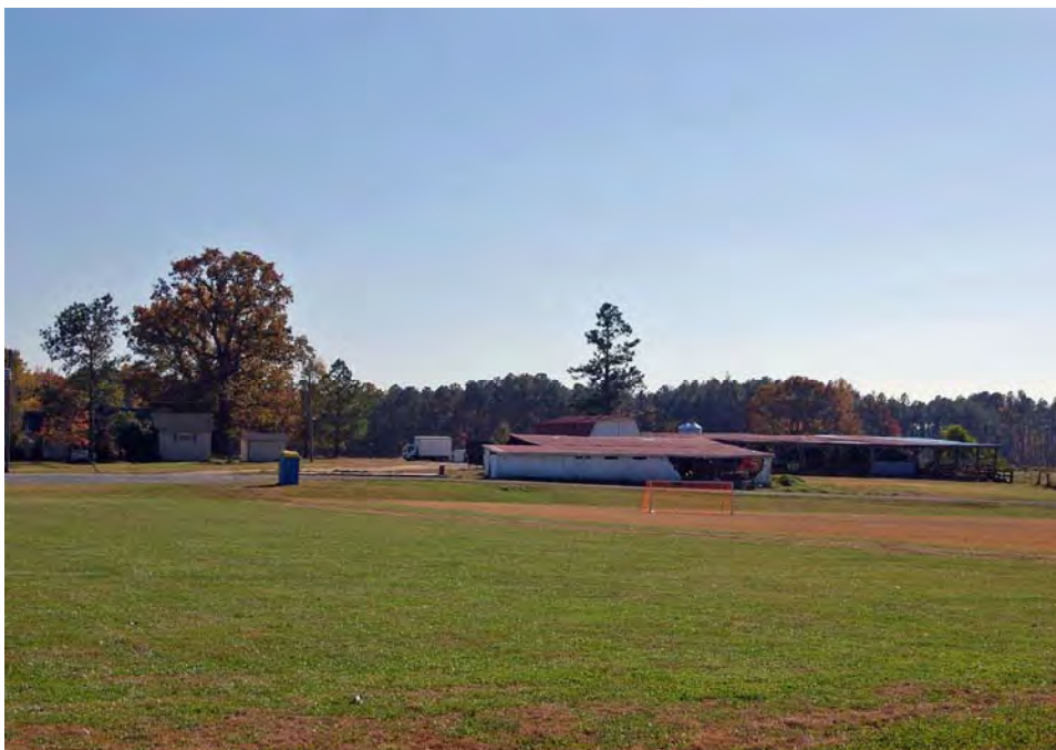
Plate 128. C. B. Sorrell House, Looking South towards Pierce Farm.
