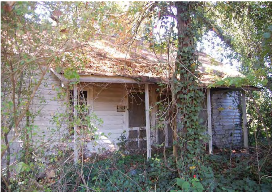
Plate 31. W. A. Gowers Farm, Tenant House, Looking Northwest.
