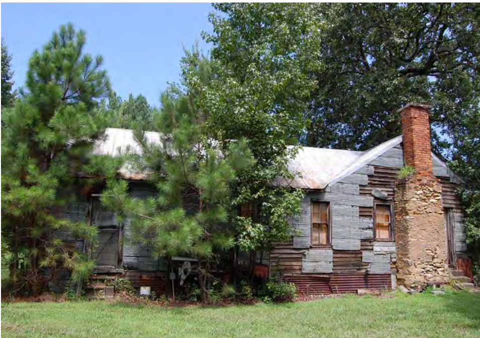
Plate 89. Wes Jones Farm, House, Side (South) Elevation, Looking North.
