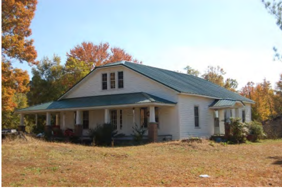
No. 196 House (PIN 1742892181), 7800 Poole Road, Garner Vicinity, Wake County
