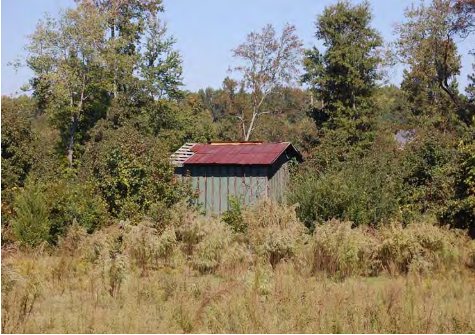
Plate 34. W. A. Gowers Farm, Tobacco Barn, West of Main Farm Complex, Looking North.
