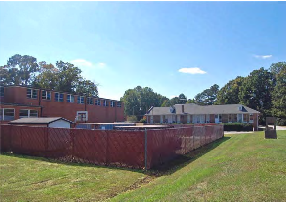
Plate 52. Mount Auburn School, Gymnasium, Rear Elevation, Looking West towards School.
