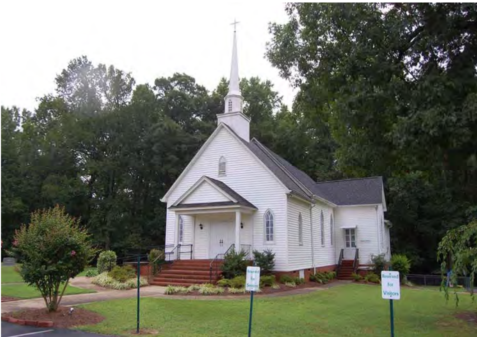
Plate 165. Wentworth Christian Church, Church and Setting, Looking South.
