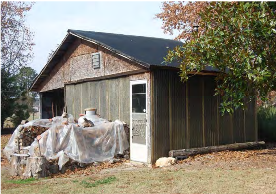
Plate 139. Bell-Pierce Farm, Eastern Tract (WA1252), Greenhouse, Looking Northwest.
