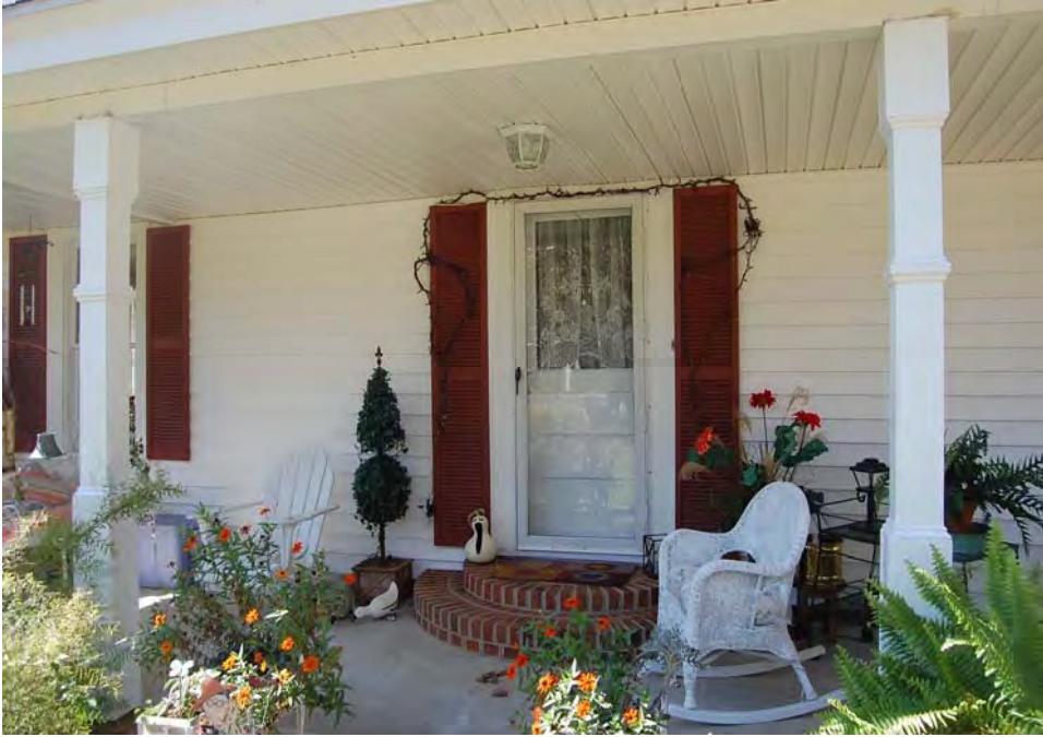
Plate 246. Juniper Level, House, 9114 Sauls Road (WA5733), Front Porch and Entrance.
