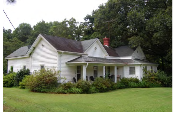
No. 28 McCullers Site 1-House (WA1219e) (PIN 0699141280), 8600 Ten Ten Road, Garner Vicinity, Wake County
