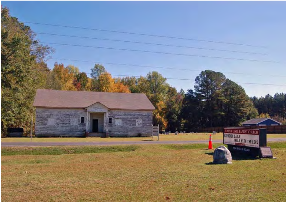
Plate 254. Juniper Level, Panther Branch School, East Side of Sauls Road, Looking East.
