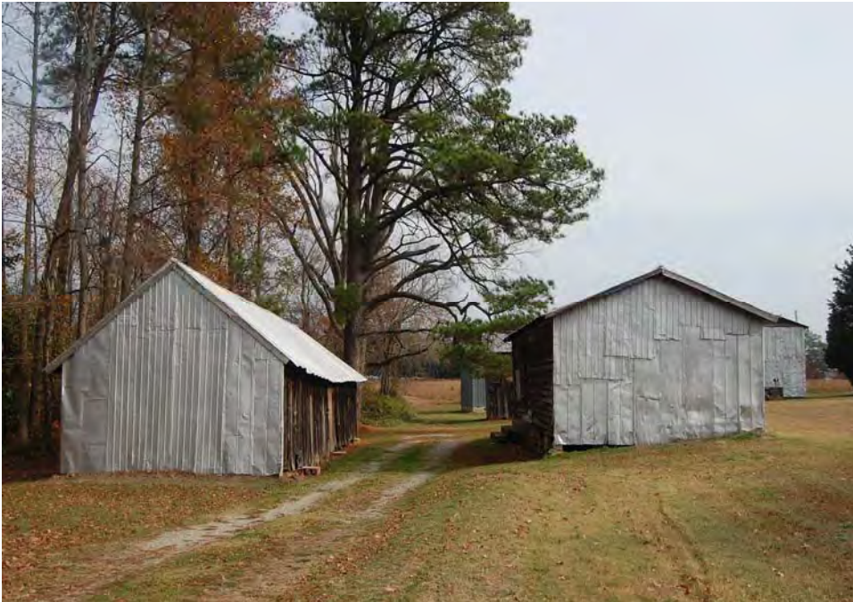
Plate 220. George Williams Farm, Packhouses, Looking East.
