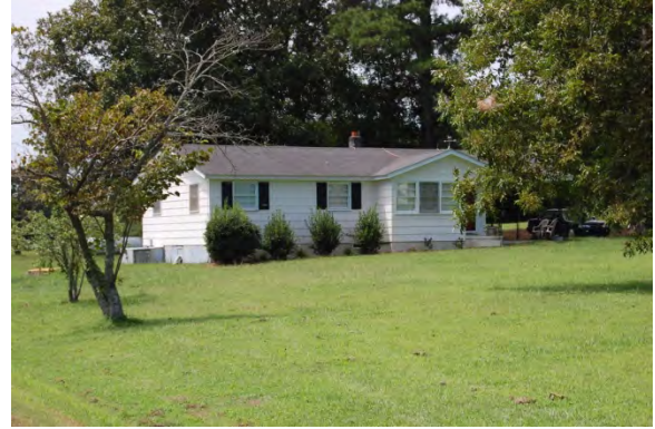
No. 21 House (PIN 0689089515), 3904 Johnson Pond Road, Apex Vicinity, Wake County
