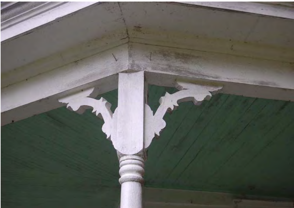
Plate 71. Baucom-Stallings House, Porch Detail.
