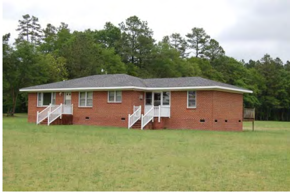
No. 157 House (PIN 1742442104) 3121 Hodge Road, Garner Vicinity, Wake County
