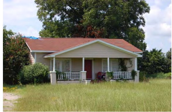
No. 50 House (PIN 1608162578), 5316 Holland Church Road, Garner Vicinity, Wake County
