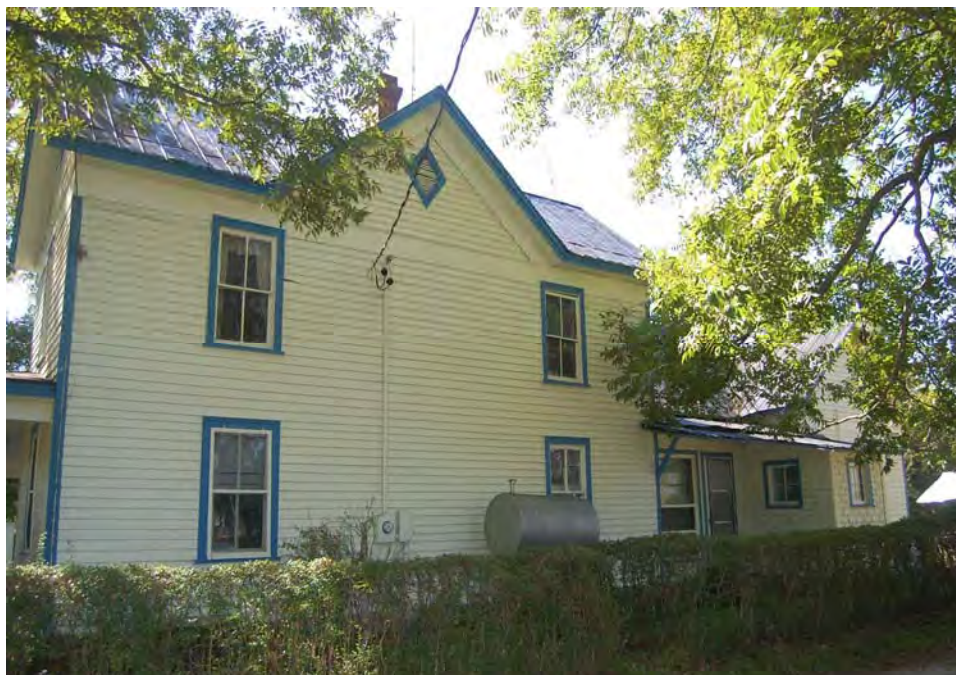
Plate 24. W. A. Gowers Farm, House, Side (North) Elevation, Looking Southwest.
