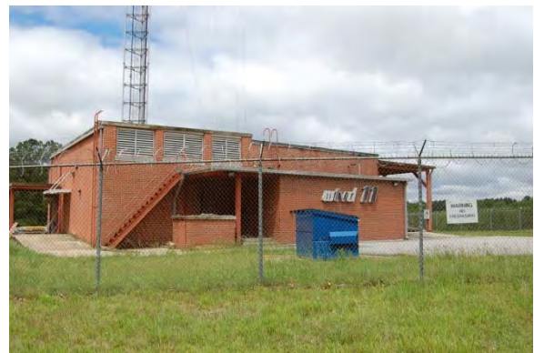
No. 154 Office and Transmitter Building (PIN 1639888459), 2901 Transmitter Road Garner Vicinity, Wake County
