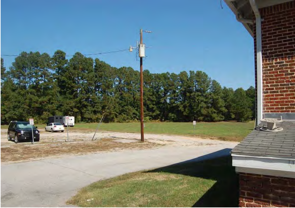
Plate 55. Mount Auburn School, Athletic Field and Parking Lot, Looking North.
