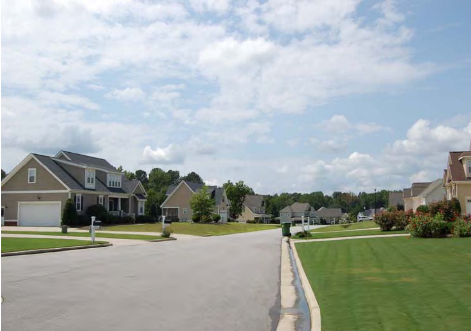
Plate 240. Juniper Level, Modern Residential Subdivision, West Side of Sauls Road, Looking West.
