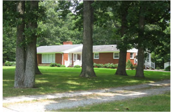
No. 183 House (PIN 0689855990), 8301 Fayetteville Road, Garner Vicinity, Wake County
