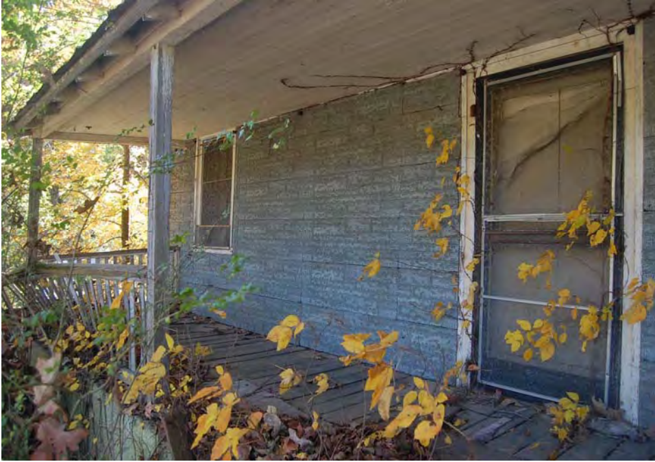
Plate 88. Wes Jones Farm, House, Front Porch and Entrance, Looking Southwest.
