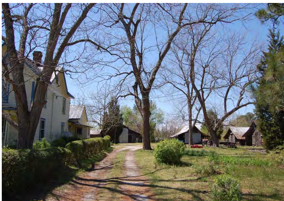
Plate 25. W. A. Gowers Farm, Outbuildings, Looking West.
