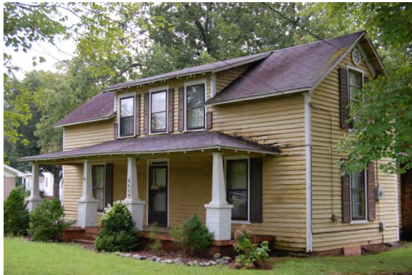
No. 29 McCullers House Site 1-House (WA1219a) (PIN 0699144356), 8604 Ten Ten Road, Garner Vicinity, Wake County
