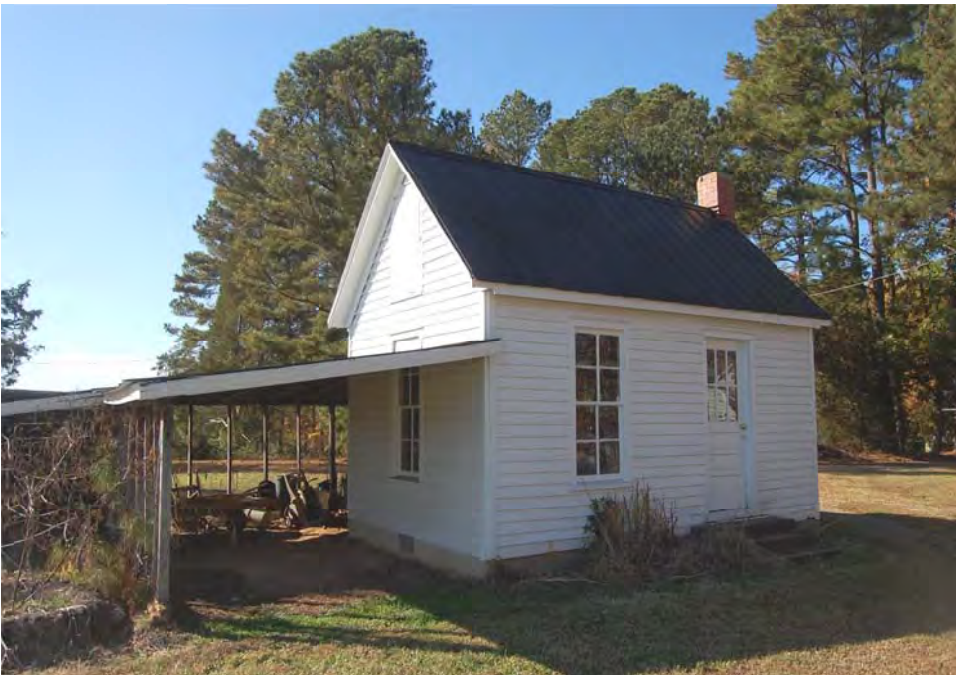
Plate 127. C. B. Sorrell House, Storage Building, Looking West.
