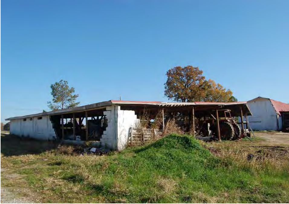
Plate 110. Pierce Farm, Former Chicken House/Equipment Storage Shed, Looking Southeast.
