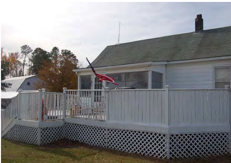
Plate 133. Bell-Pierce Farm, Eastern Tract (WA1252), Bell-Pierce House, Rear Deck, Looking West.
