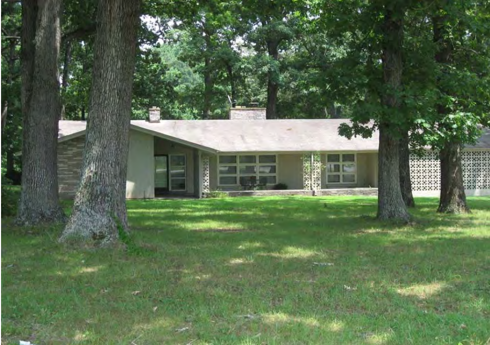
Plate 367. Gerald Cochran House, House and Setting, Looking East.
