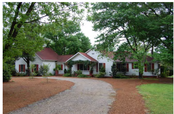
No. 146 John Robert Baucom Farm (WA2250) (PIN 1741609431), 7920 Old Baucom Road Garner Vicinity, Wake County
