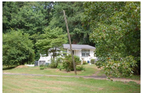
No. 5 House (PIN 0669098920), 9628 Holly Springs Road, Holly Springs, Wake County
