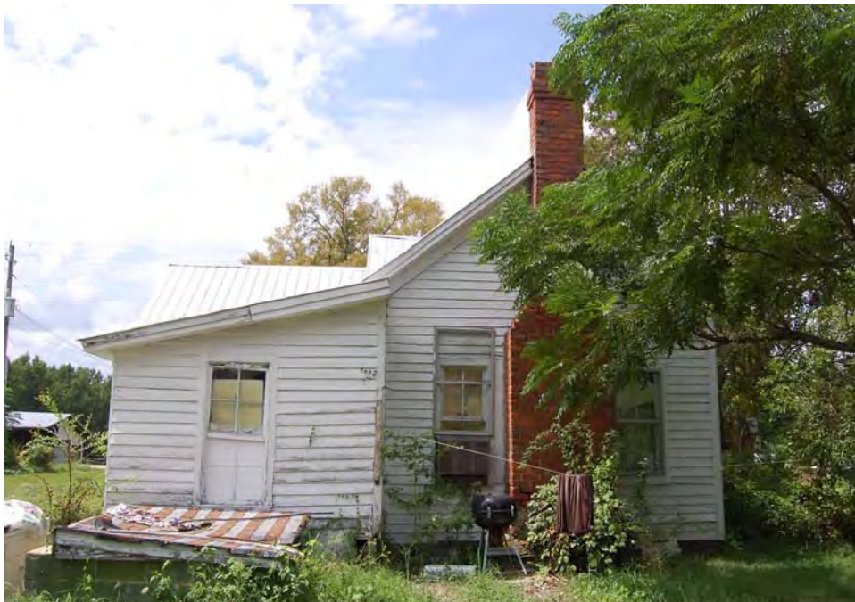
Plate 271. Jones Family Farm, House, Rear Elevation of Rear Ell, Looking West.
