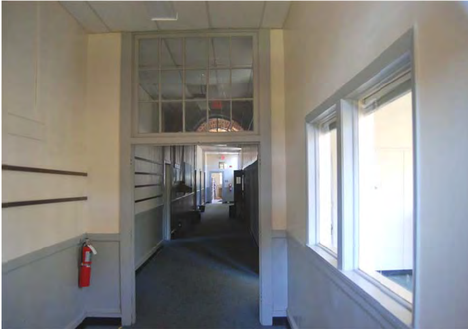
Plate 49. Mount Auburn School, Hallway, Looking into North Wing from West Entrance.
