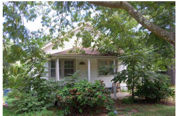
No. 17 House (PIN 0679690742), 8101 Bells Lake Road, Apex Vicinity, Wake County
