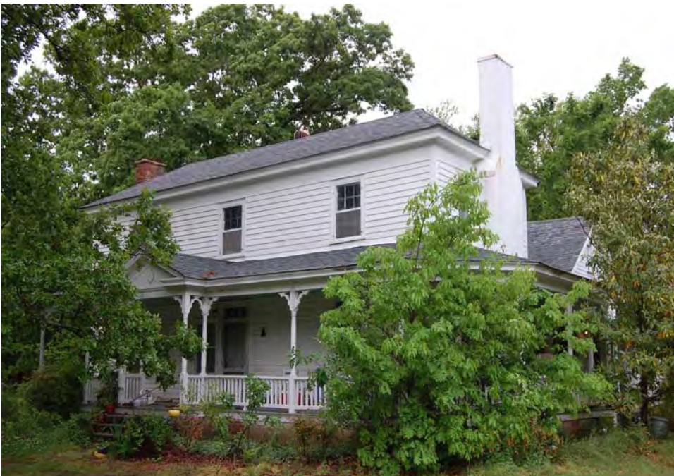
Plate 69. Baucom-Stallings House, Façade (South Elevation), Looking North.
