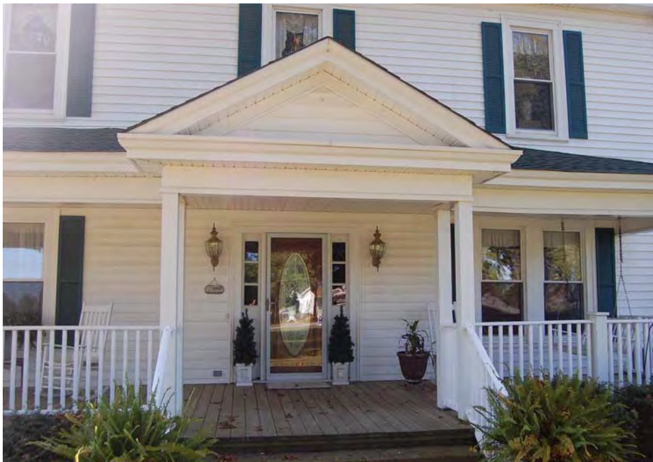
Plate 233. Samuel Jefferson Rhodes House, Entrance, Looking West.
