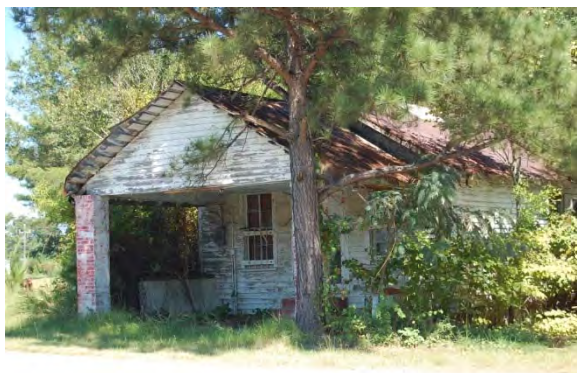
No. 77 Store (PIN 163802-77-4585), 6859 Cornwallis Road, Clayton Vicinity, Johnston County
