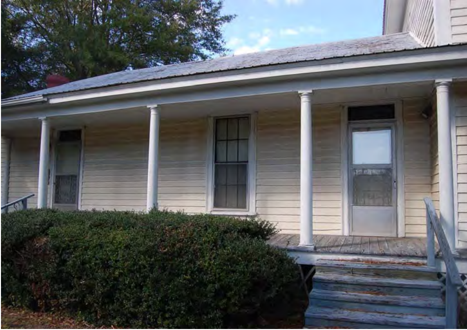
Plate 14. John B. Strain House, Rear Porch, South Elevation, Looking North.
