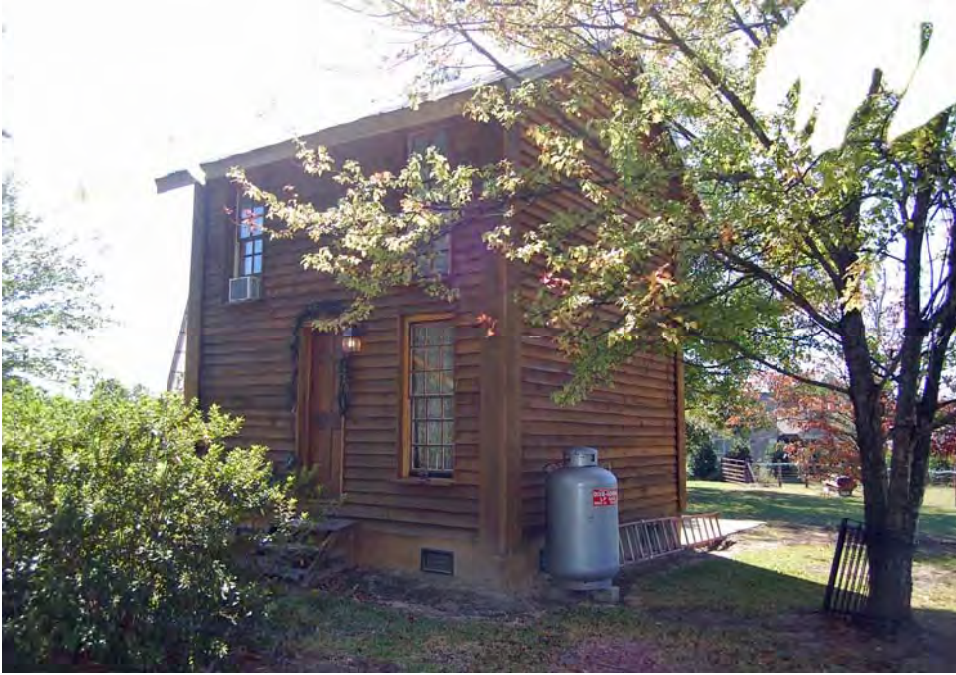
Plate 250. Juniper Level, House, 9114 Sauls Road (WA5733), Modern Other House, Looking West.
