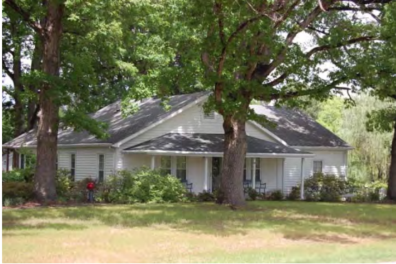
No. 163 House (PIN 1743307176) 7317 Poole Road, Garner Vicinity, Wake County
