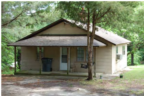
No. 161 House (PIN 1742376932) 2737 Hodge Road, Garner Vicinity, Wake County
