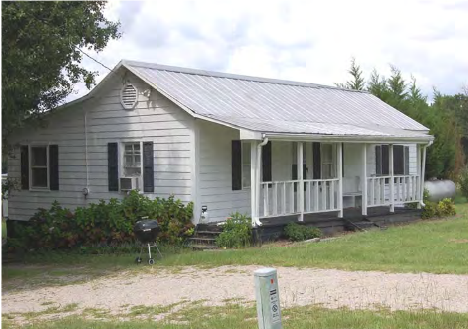
Plate 280. Jones Family Farm, Second House (No. 59) on West Side of Jordan Road, Looking West.
