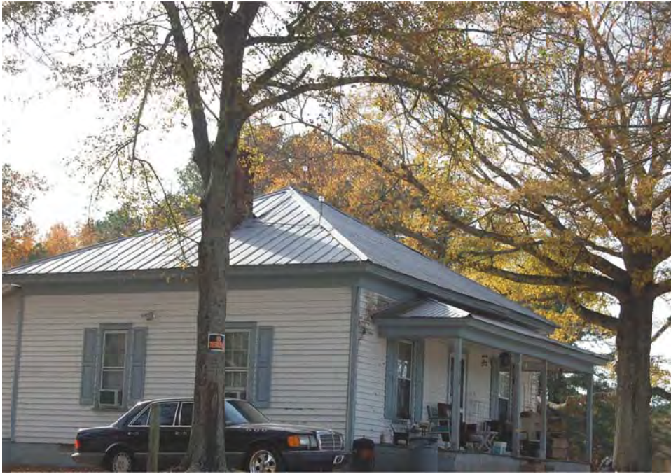
Plate 206. Williams Crossroads, Hip-Roofed Dwelling (WA1218) (Outside APE) on South Side of Ten Ten Road, Looking West.
