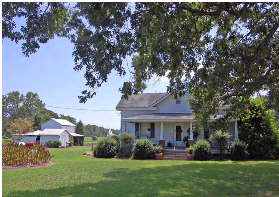
Plate 130. Bell-Pierce Farm, Eastern Tract (WA1252), Bell-Pierce House and Outbuildings, Looking South.
