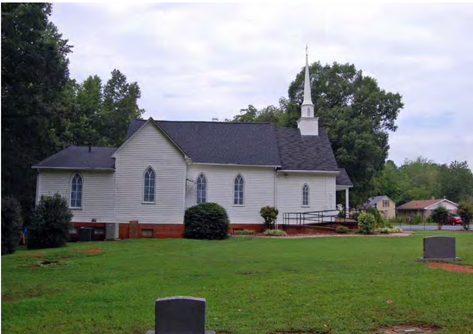
Plate 167. Wentworth Christian Church, Side (East) Elevation, Looking West.
