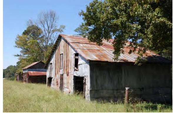
No. 79 Farm Complex (PIN 163800-43-8740), 719 New Bethel Road, Clayton Vicinity, Johnston County
