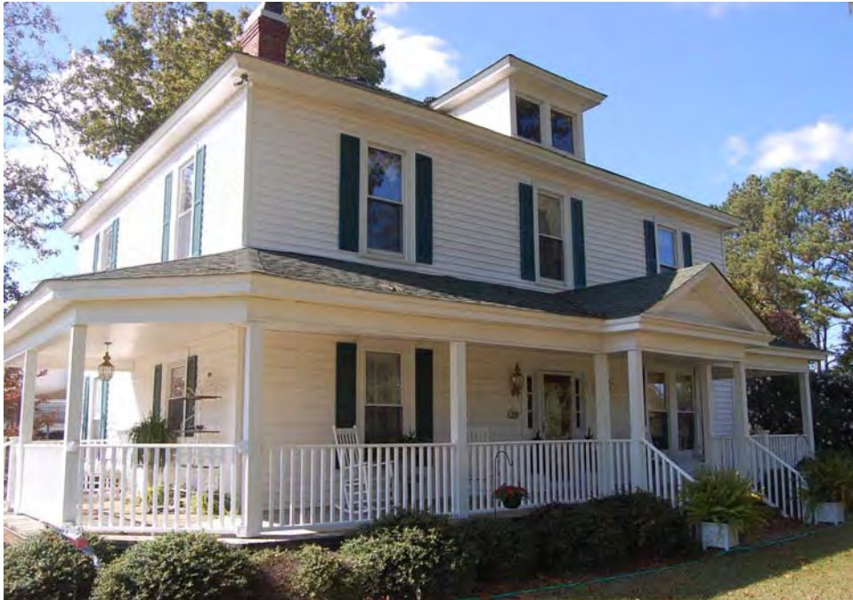
Plate 231. Samuel Jefferson Rhodes House, Façade, Looking Northwest.
